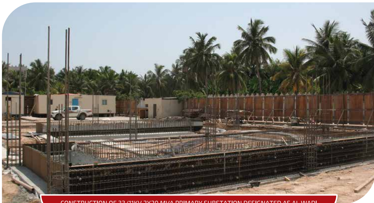
CONSTRUCTION OF 33/11KV,2X20 MVA PRIMARY SUBSTATION DESIGNATED AS AL WADI
