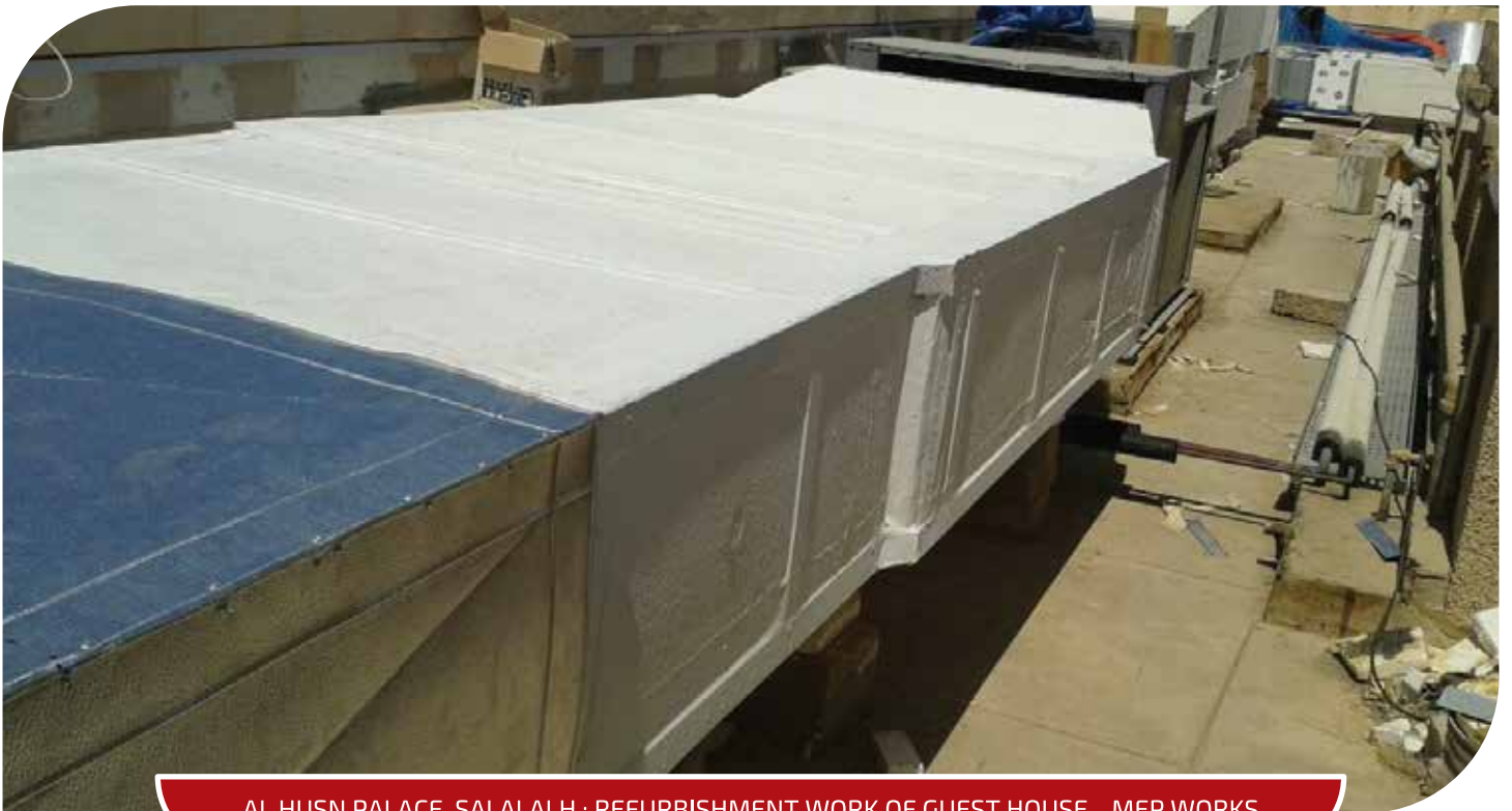
AL HUSN PALACE, SALALAH : REFURBISHMENT WORK OF GUEST HOUSE - MEP WORKS
