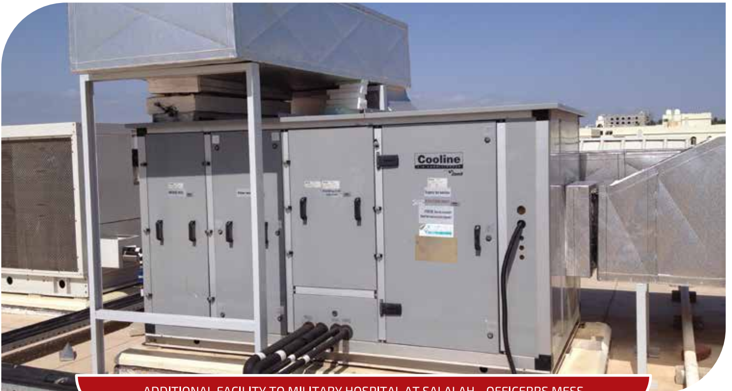
ADDITIONAL FACILITY TO MILITARY HOSPITAL AT SALALAH - OFFICERS MESS
